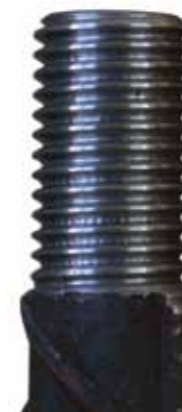
Threads on a non-upsetted rebar.
